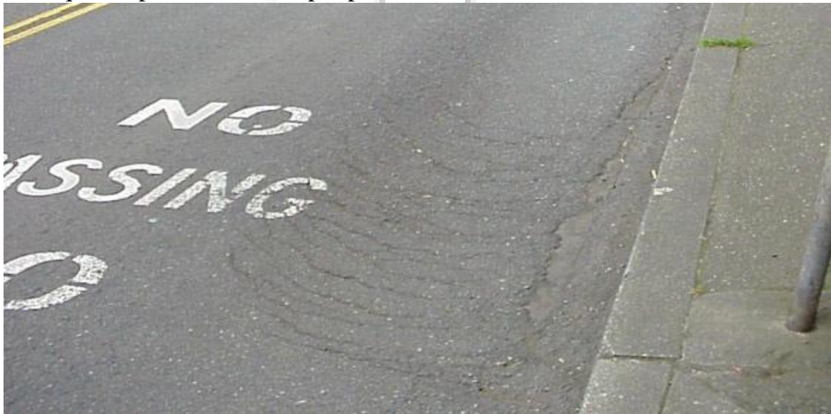
Fig. Slippage Cracks
