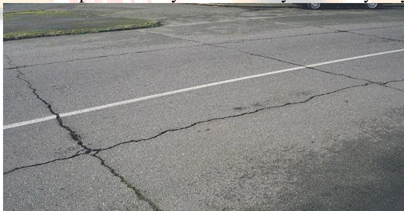
Fig. Joint Reflection Cracks
