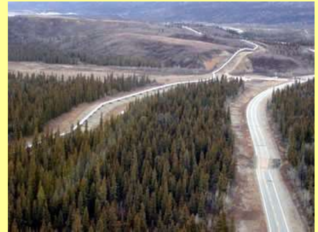
Aerial view of the Trans-Alaska Pipeline and Richardson Highway. Rupture along the fault resulted in displacement of the highway. Photo by Patty Crow, DGGS.
