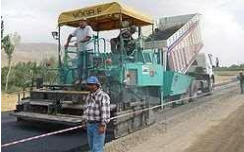
Fig. Road Paver
