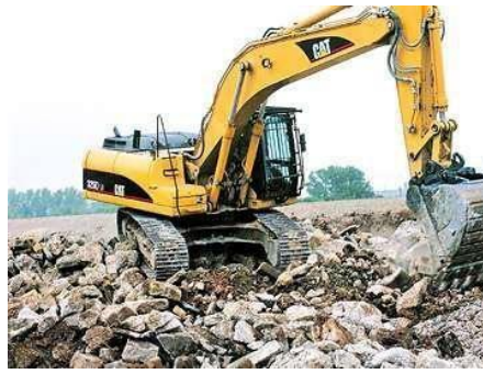
Fig. New Power Shovel
