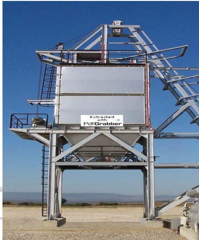
Fig.Hot mix storage silo
