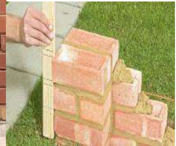
45. Brickwork Gauge Rod
