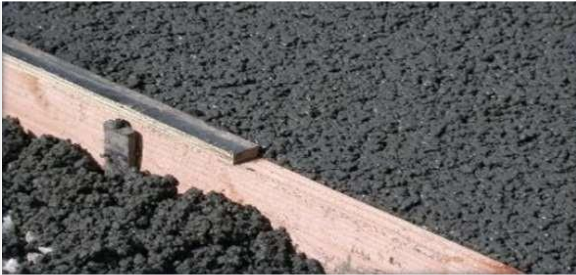
Fig-7 No Fines Concrete
