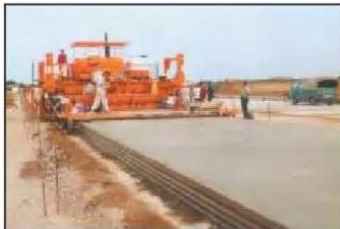
Fig-6 placing of concrete
